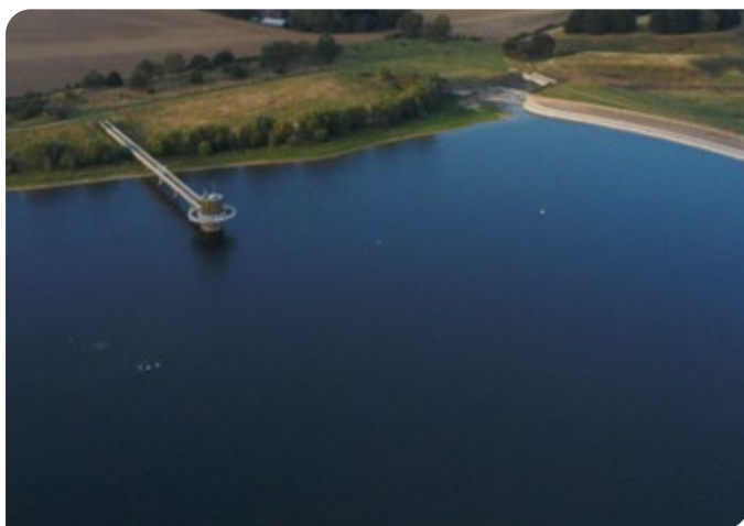
Figure 1: Anglian Water's Alton Water Reservoir and treatment works treat up to 10 million Imperial gallons of water a day.
