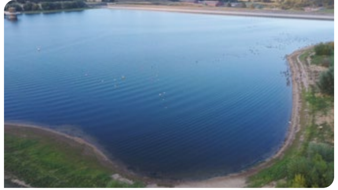
Figure 3: The Alton WTW supplies water to 92,214 properties in the Suffolk area, United Kingdom.
